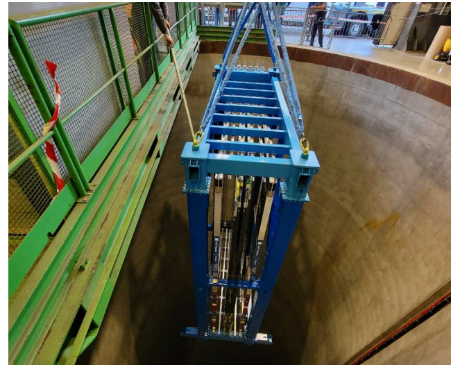
Lowering of part of the Scintillating Fibre detector into the LHCb cavern (Photo: Blake Leverington).
