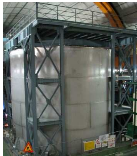
Figure 3.1: The GERDA water tank for the Cerenkov shield and the superstructure during its installation.
