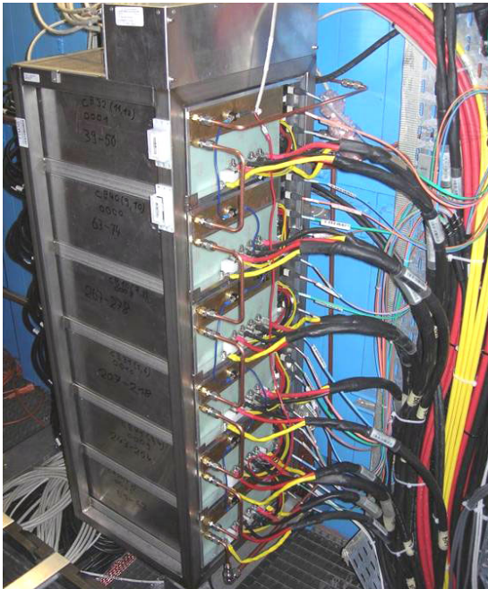
Figure 16.1: Part of the readout electronics of the LHCb trigger tracker.
